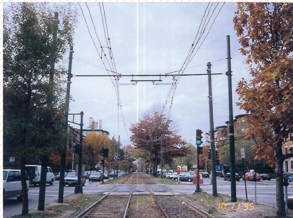
Rebuilt Overlaps
