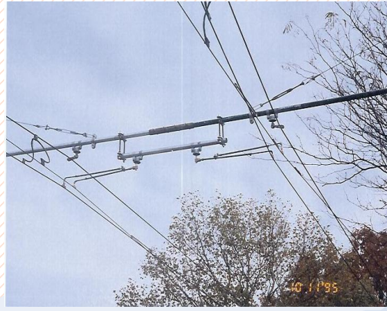
Rebuilt Overlaps
