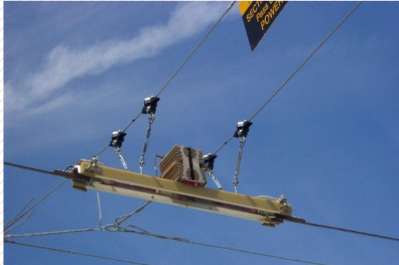
Diode section insulator
