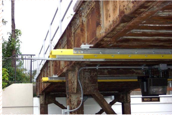
Low bridge supports
