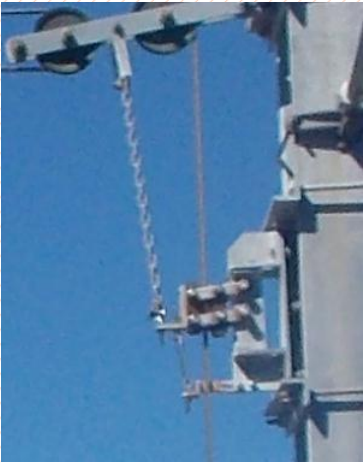
Balance Weight Brake
