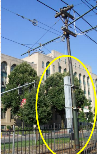
Between the Tracks Balance Weight
