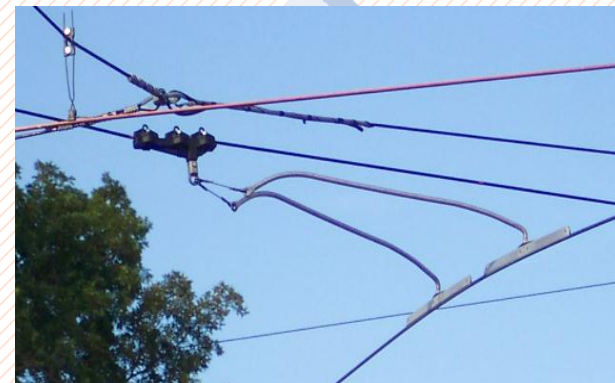
Pole/pantograph curve pullovers
