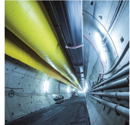
T4 Fréjus Tunnel: construction of Safety Tunnel
