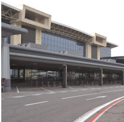
Construction of aprons, service roads, extension of terminal Milan Malpensa Airport - Terminal 1
