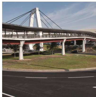
Underground structures and construction of connecting walkway Milan Malpensa Airport - Terminal 1
