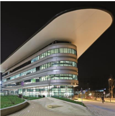
University of Turin: construction of new campus – Faculty of Law and Political Science
