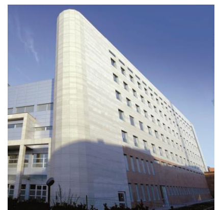
Expansion of General Hospital in San Donato Milanese (Milan)
