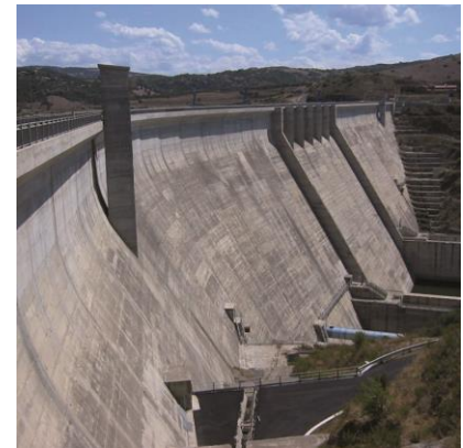
Sardinia: Construction of a dam on Tirso river
