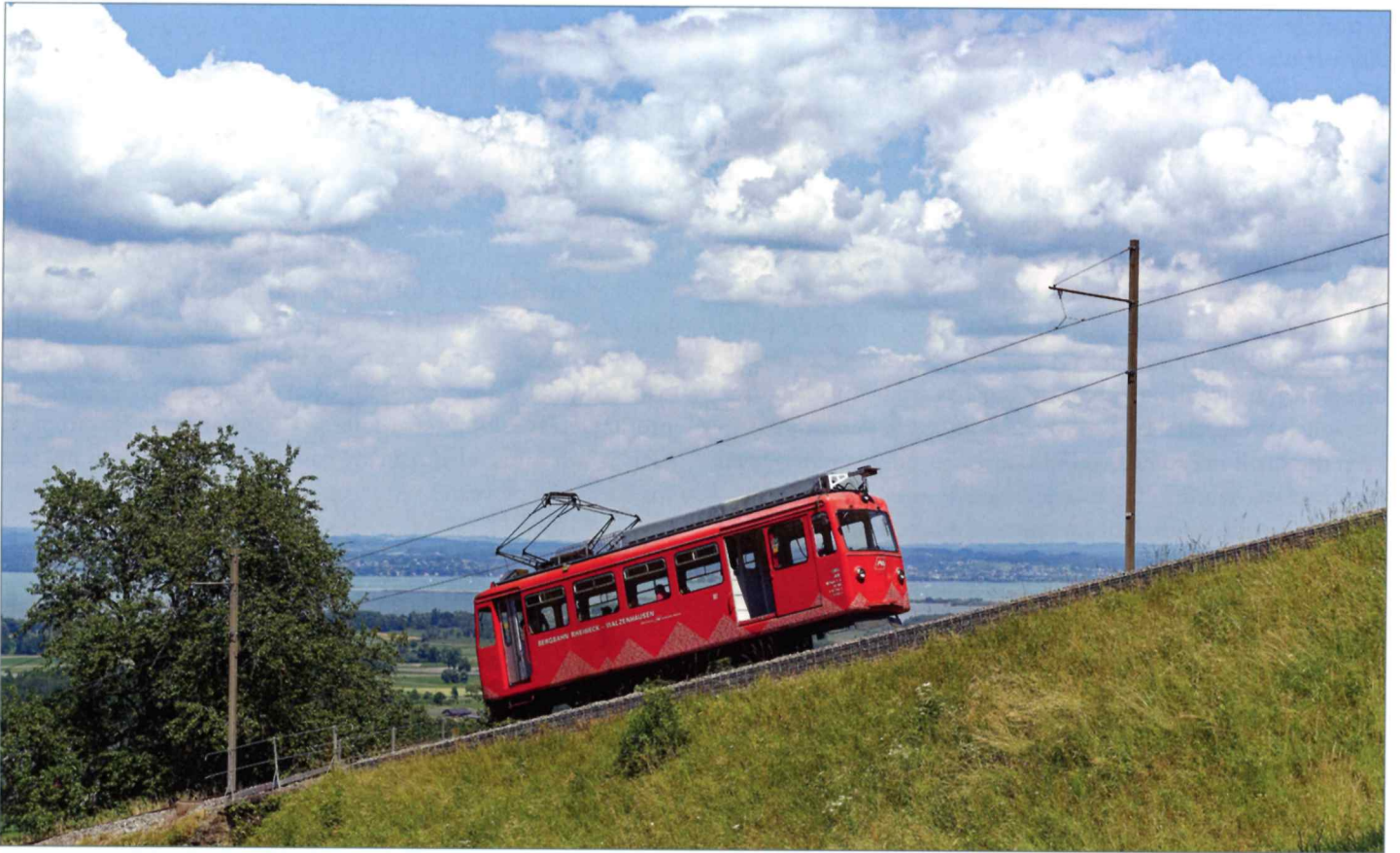
Between Rheineck and Walzenhausen the maximum gradient is 253‰ (1 in 3.95). In Switzerland, there is only one rack railway that is even steeper, the Pilatus Railway, equipped with the unique Locher rack system, with a maximum of 480‰ (1 in 2.08). The railcar is descending to Rheineck on 15 June 2023.
