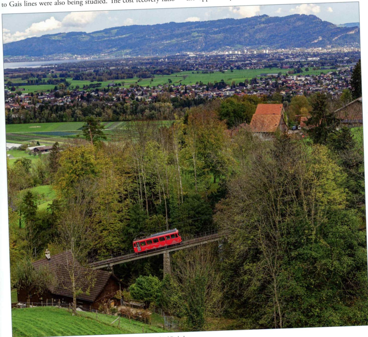
On 4 November 2022, the railcar crosses the bridge over the Hexenkirchlitobel.
