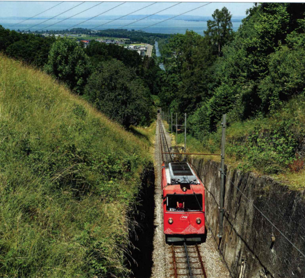
On 15 June 2023, with the Schutz tunnel in the distance the railcar is about to pass under the overbridge shortly before the Walzenhausen tunnel to the terminus. Between Ruderbach and Walzenhausen the track is a continuous straight. In the upper section of the line, modern von Roll racks have been installed. Today, Riggenbach racks are only in the lowest section.
