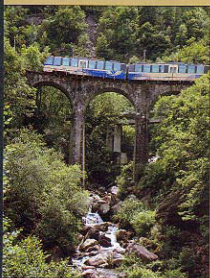
New Centovalli EMU 082 crossing a viaduct near Trontano, while forming a special train to Santa Maria Maggiore.
